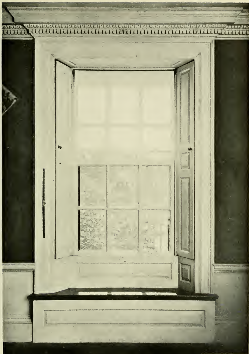
PLATE CII.—Detail of Embrasured Window and Seat, West Parlor, Pierce-Johonnot-Nichols House.
